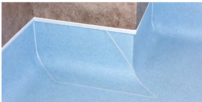
Figure 3.9 External corners 'wrap around method'
