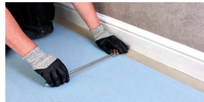
Figure 3.2 Scribing the wall profile
