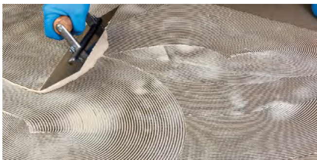
Figure 3.6 Spread the adhesive
